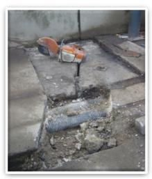
Figure 11 - Ducts in Bridge Deck
